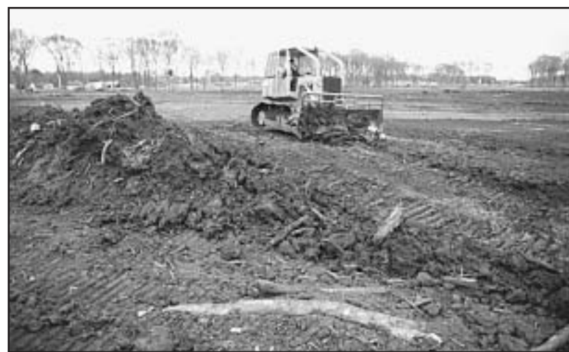
MARCH 1, 1996: Ground-breaking begins
