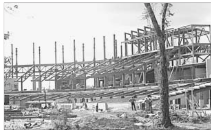
DEC. 11, 1996: A stadium is shaped
