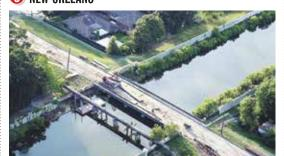
The Filmore Avenue bridge over the London Avenue Canal is being replaced with a new span with floodwalls. Until its completion, only sandbags will stop hurricane surge from pouring into city neighborhoods.
