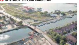
The Hammond Highway bridge over the 17th Street Canal is being replaced with a new, hurricane-resistant structure. Huge sandbags are kept nearby to plug this hole in the hurricane protection for Jefferson and Orleans parishes
