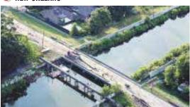
The Filmore Avenue bridge over the London Avenue Canal is being replaced with a new span with floodwalls. Until its completion, only sandbags will stop hurricane surge from pouring into city neighborhoods.
